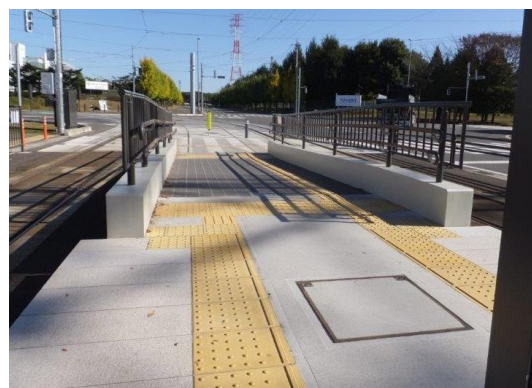
The slope of the platform
