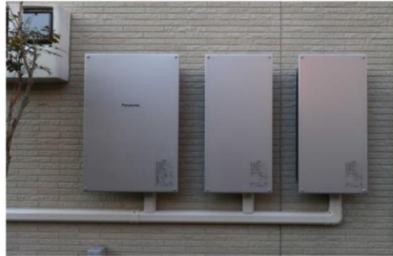
Related devices: Power conditioner (left) & Converters for storage batteries
